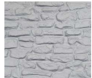
Rubble Stone Wall
